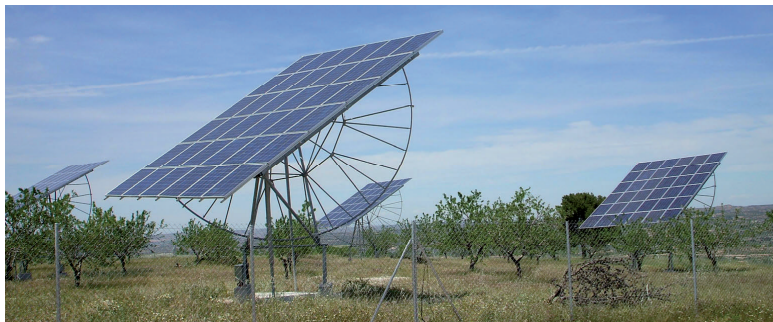
Image 1: TETRA-TRACK® installation
