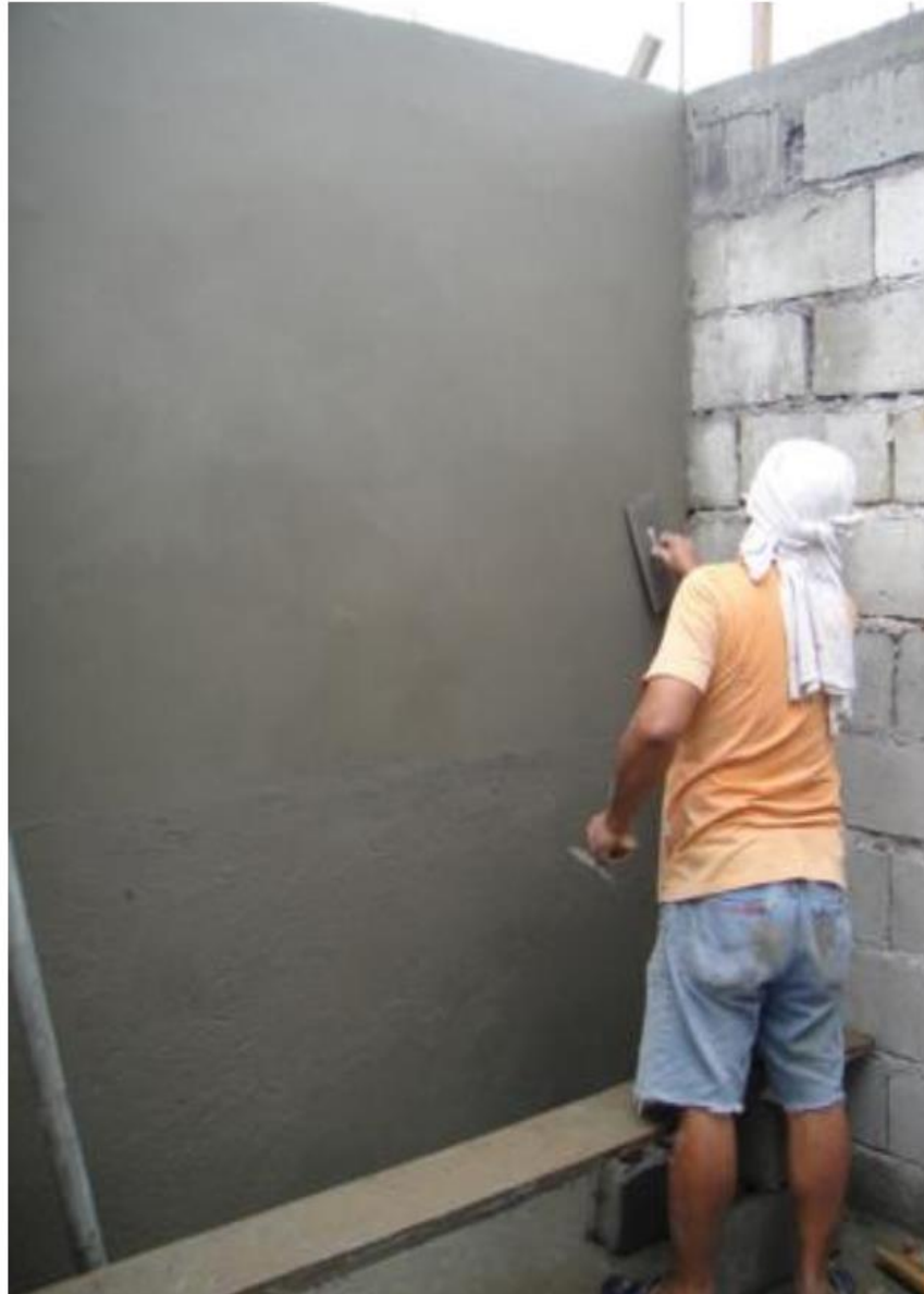
Fig. Wall Cement mortar plastering
