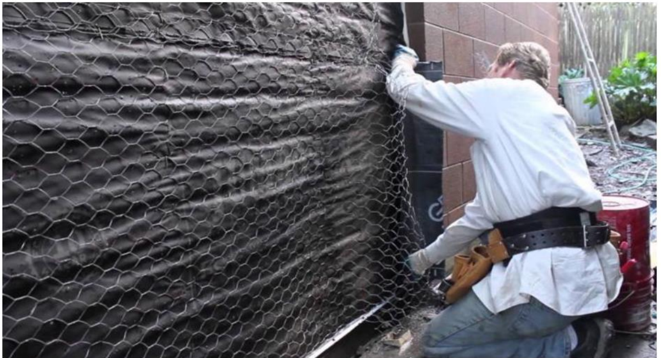
Fig. Water proofing plastering
