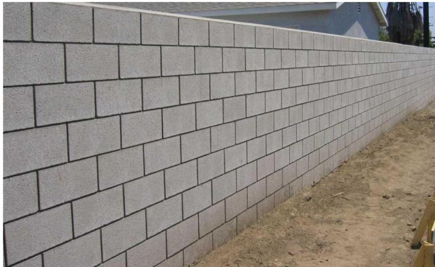
Concrete blocks wall
