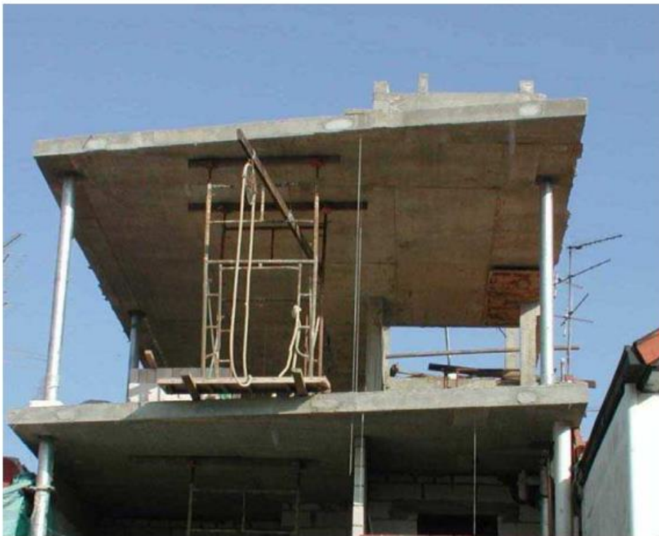
Flat plate system with circular steel column
