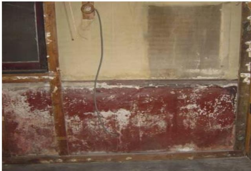
Fig. Efflorescence
