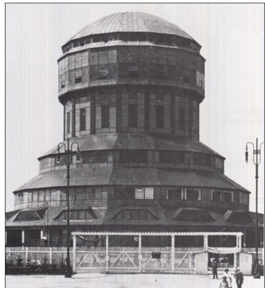
Water Tower, Posen 8
