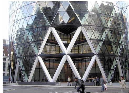
Diagrid system in "The Gherkin" 11
