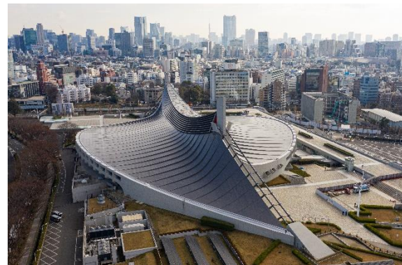
Yoyogi National Gymnasium (1964) 16
