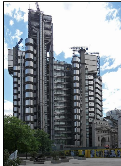
Lloyds Building (London), 1984 8
