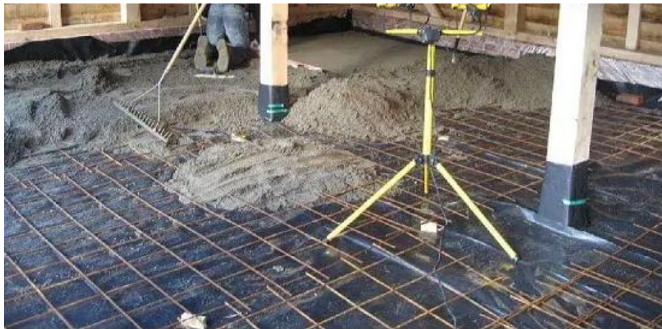
Figure: Membrane Damp Proofing
