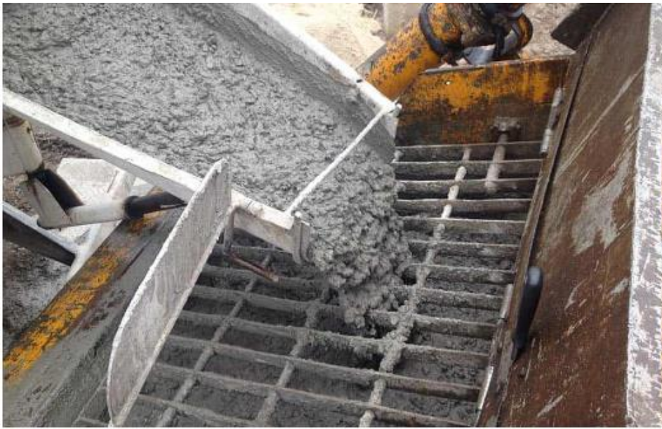
Figure: Waterproof Concrete
