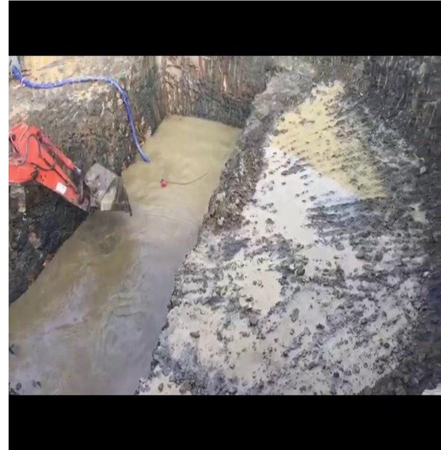
Figure: Wet Excavation
