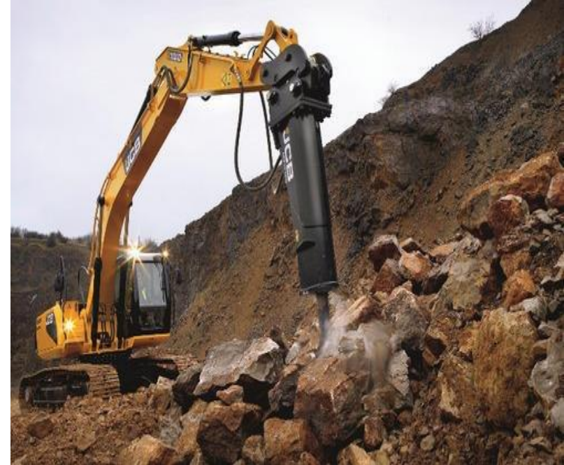
Figure: Hard rock Excavation
