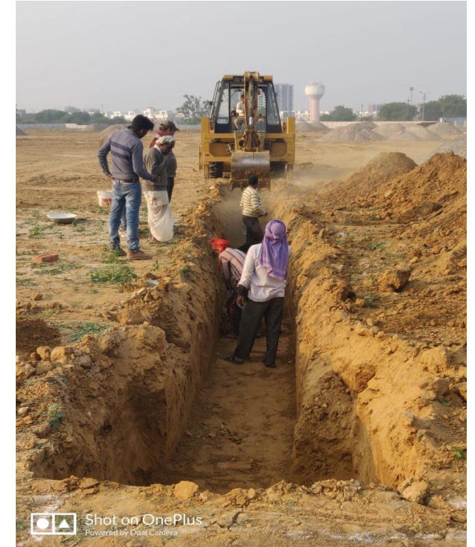
Figure: Soft Soil Excavation
