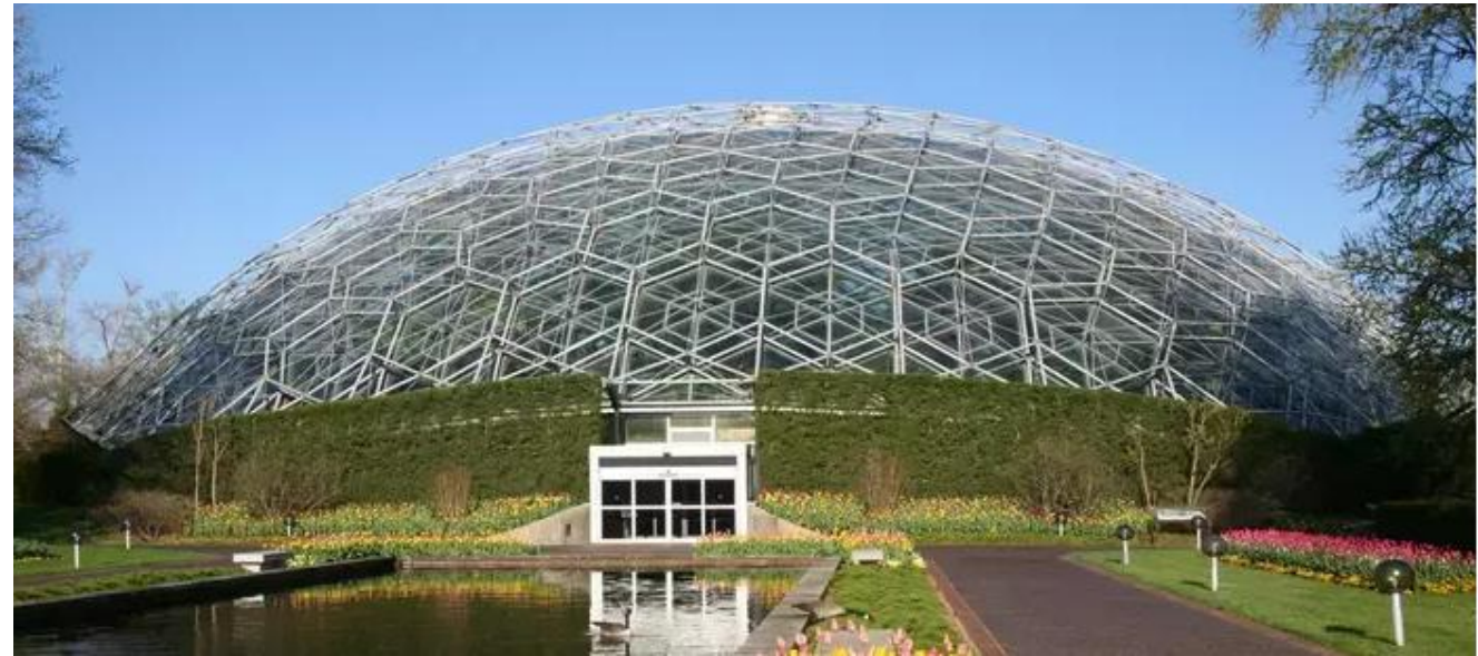
Figure : Shell roof( source: Sharma, 2023:Online) https://www.novatr.com/blog/shell-structures
