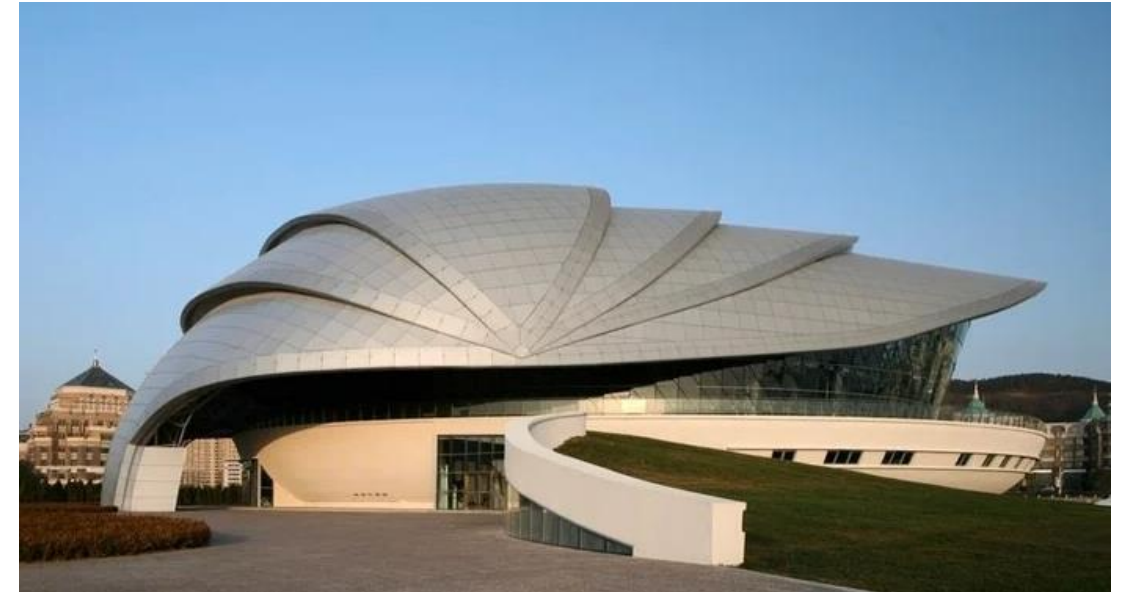
Figure : Shell roof( source: Sharma, 2023:Online) https://www.novatr.com/blog/shell-structures
