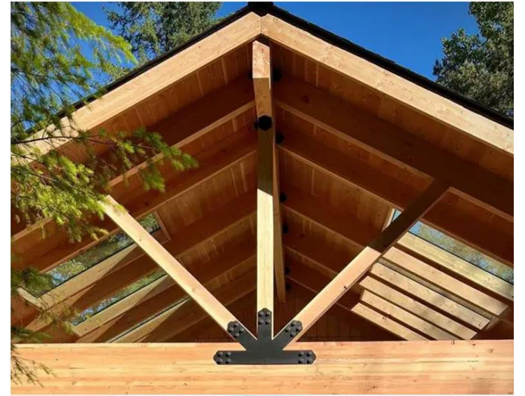
Figure: Timber truss(Source:Obinna, 2018:Online) https://structville.com/2018/04/design-of-timber-roof-truss-to-british-code.html
