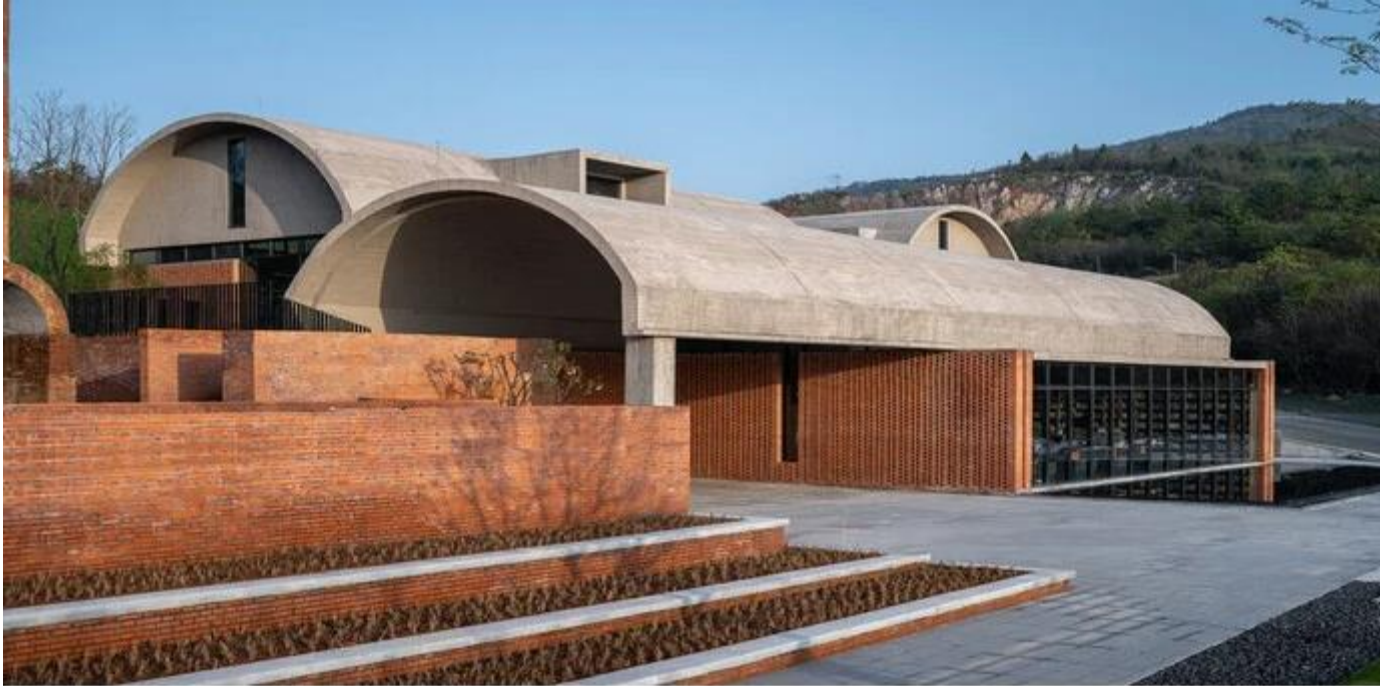
Figure : Shell roof( source: Sharma, 2023:Online) https://www.novatr.com/blog/shell-structures
