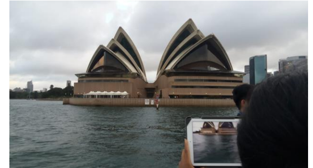
Figure: shell roof
