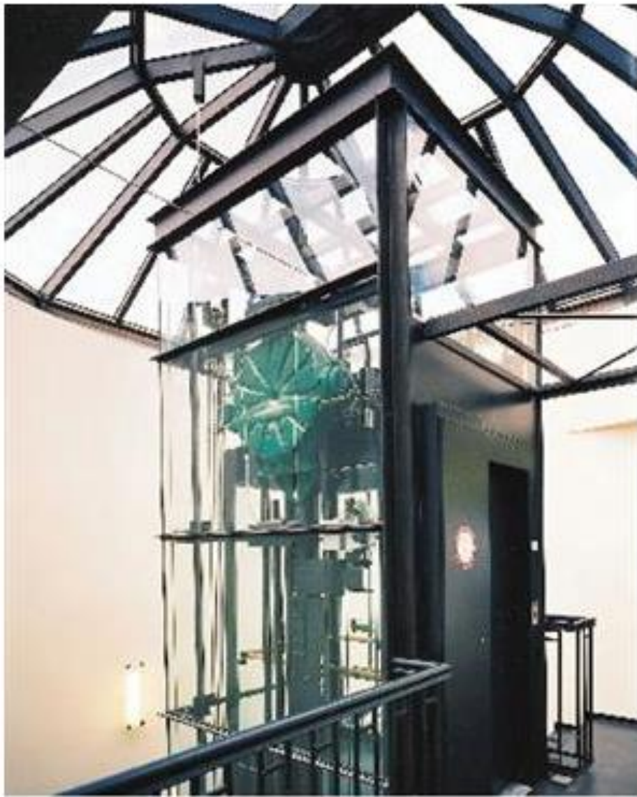
Cable Driven Elevator
