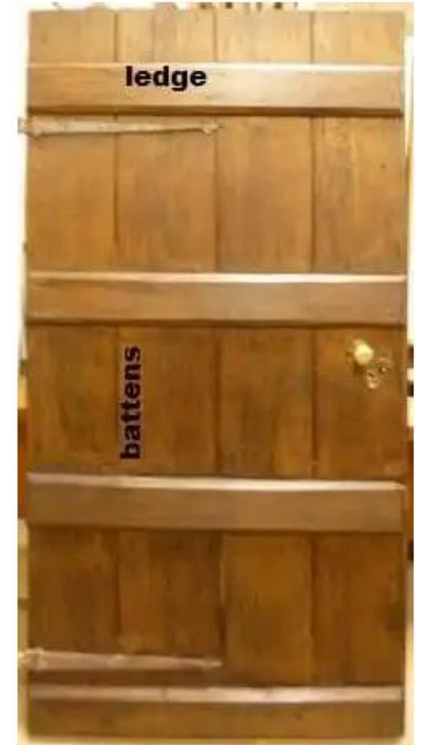
Figure: Battened and ledged door(Source: The Constructor: Building ideas. (n.d.). Retrieved from
