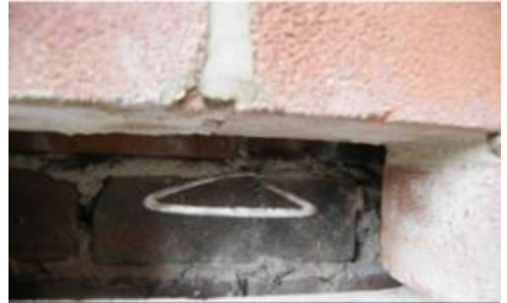
Exposed butterfly wall ties in a good condition
