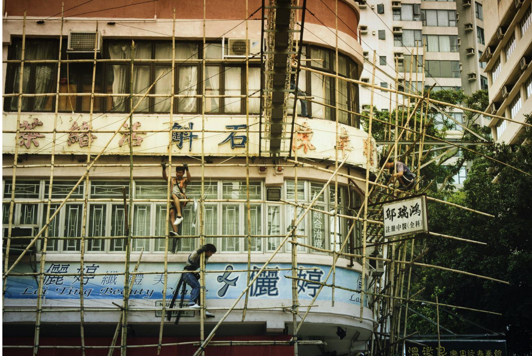
Figure: Scaffolding(source: Yakubu, P. 2023, June 23:Online), https://www.archdaily.com/1003231/the-architectural-language-of-scaffoldings-in-cityscapes-exploring-the-impact-of-these-temporary-structures
