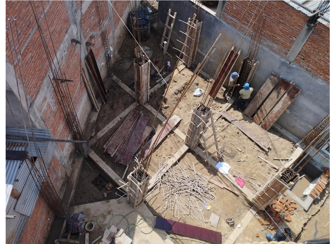
Figure: Formwork
