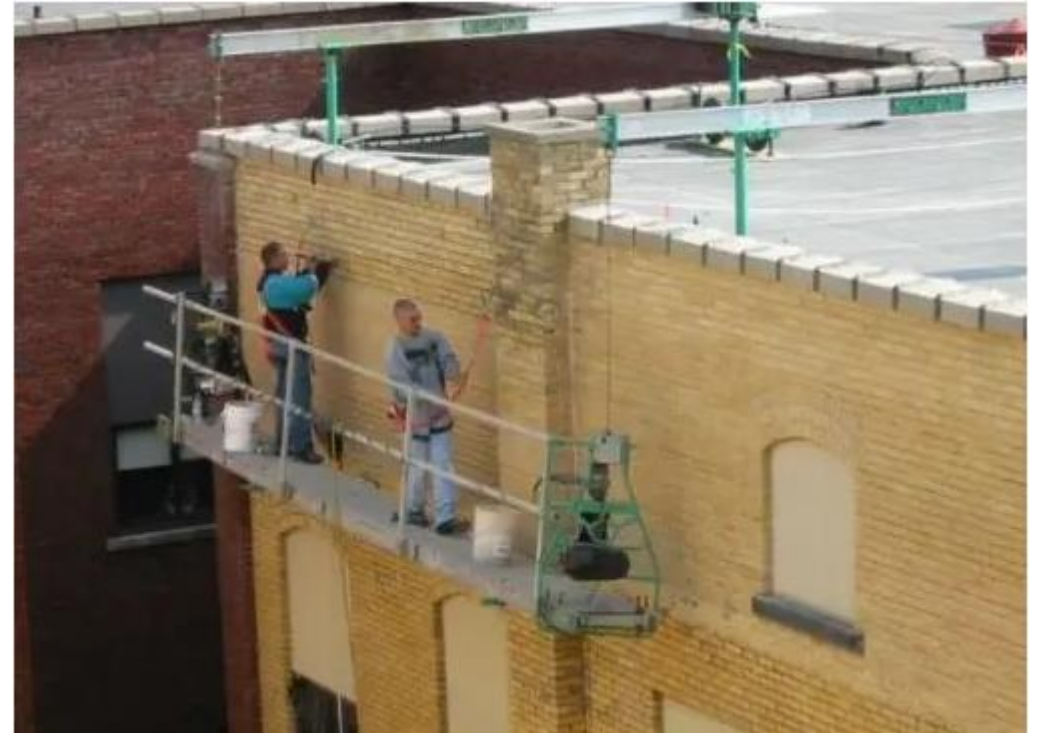
Figure: Scaffolding(source: The Constructor:Building ideas , n.d:Online), https://theconstructor.org/building/types-of-scaffolding-in-construction/11845/
