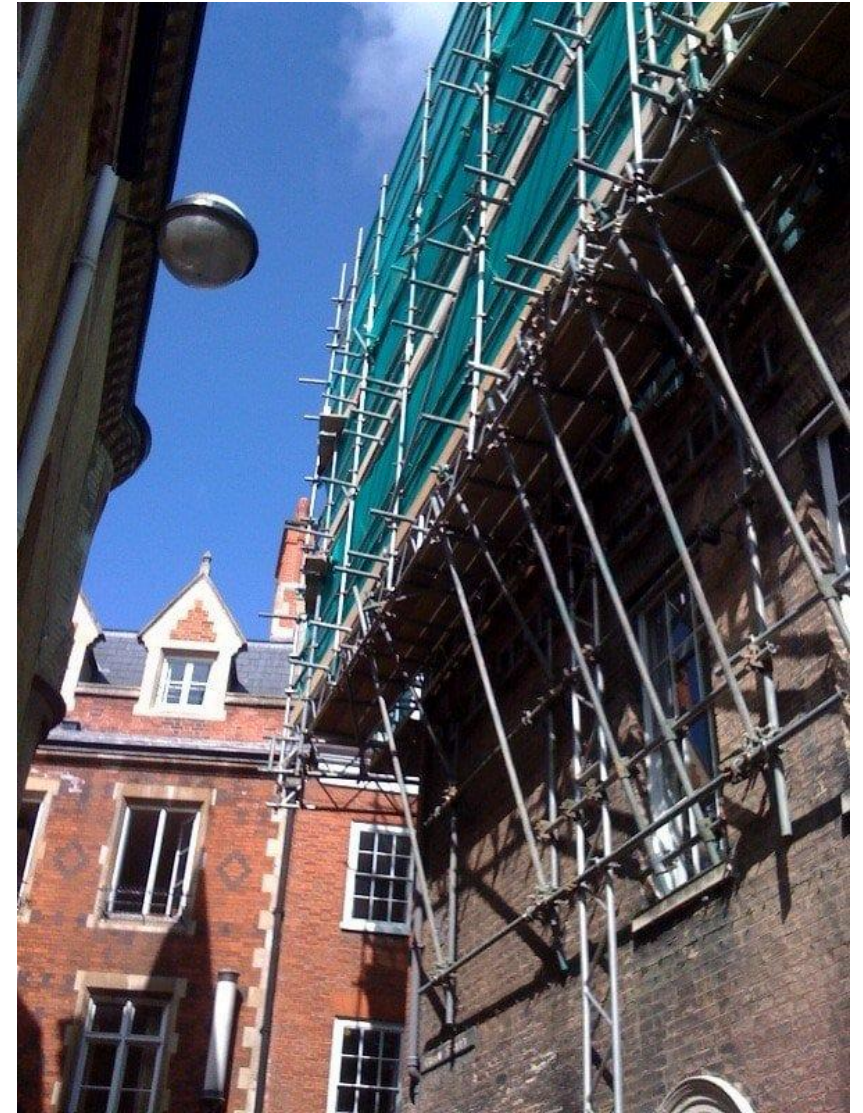
Figure: Scaffolding(source: The Constructor:Building ideas , n.d:Online), https://theconstructor.org/building/types-of-scaffolding-in-construction/11845/
