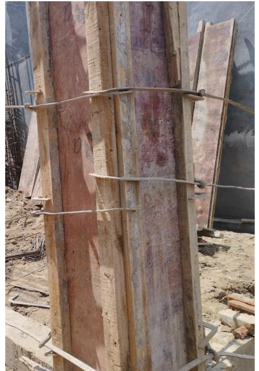
Figure: Formwork
