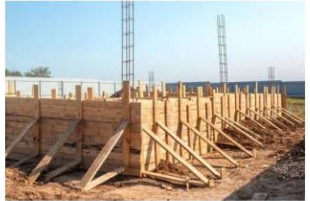
Figure: Timber Formwork (Source: testbook. (May 10, 2023). Retrieved from testbook.com:
