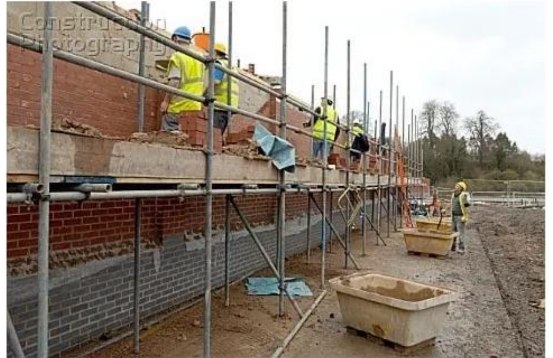
Figure: Scaffolding(source: The Constructor:Building ideas , n.d:Online), https://theconstructor.org/building/types-of-scaffolding-in-construction/11845/
