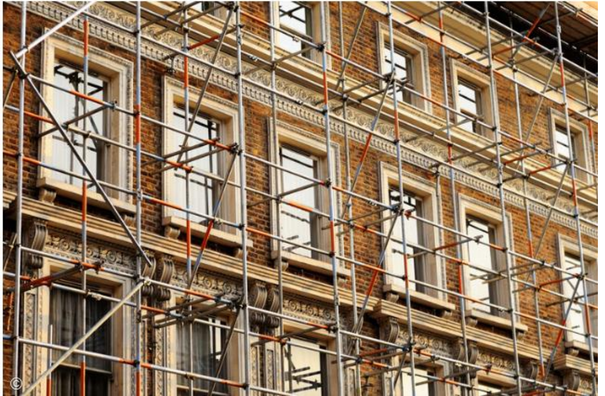
Figure: Scaffolding(source: Yakubu , P. 2023, June 23:Online), https://www.archdaily.com/1003231/the-architectural-language-of-scaffoldings-in-cityscapes-exploring-the-impact-of-these-temporary-structures
