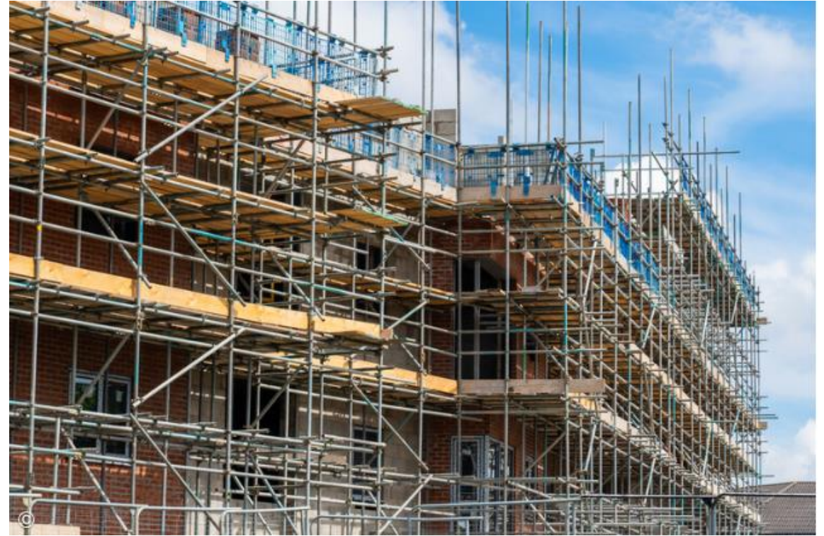
Figure: Scaffolding(source: Yakubu , P. 2023, June 23:Online), https://www.archdaily.com/1003231/the-architectural-language-of-scaffoldings-in-cityscapes-exploring-the-impact-of-these-temporary-structures
