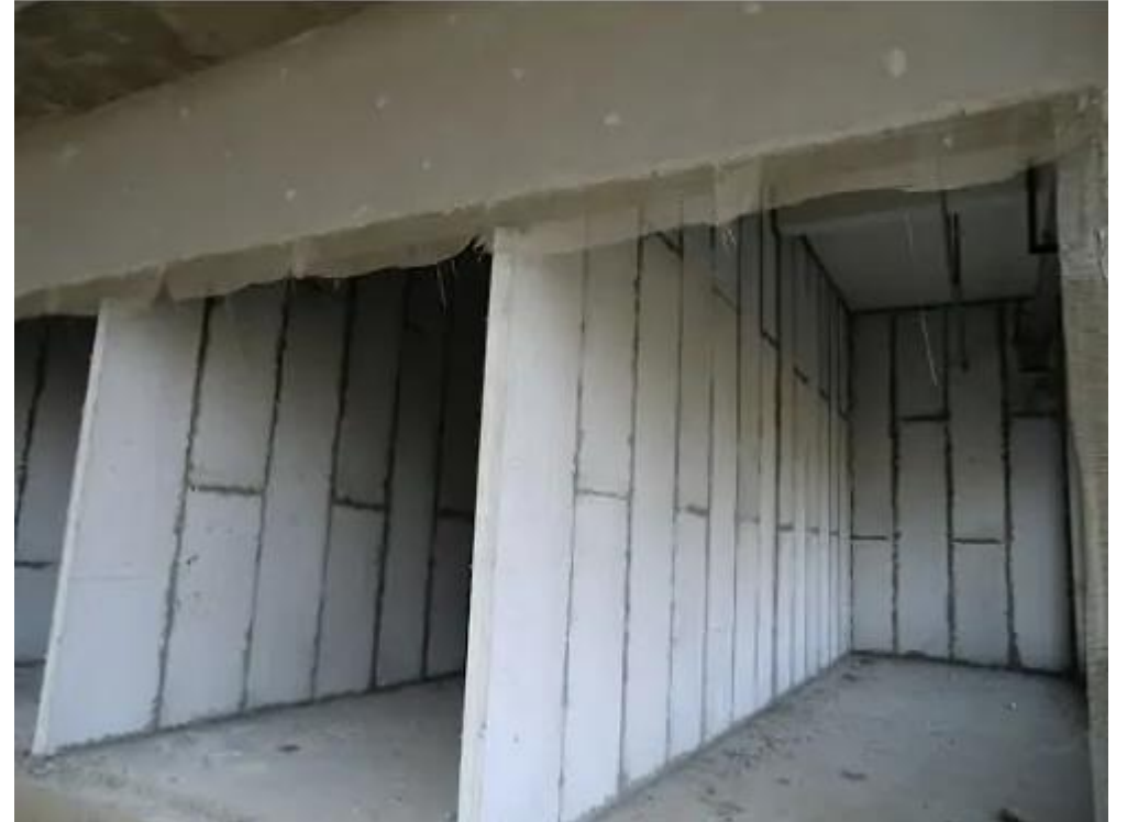
Figure: Concrete partitions(Source: Daily Civil(n.d):Online) https://dailycivil.com/partition-wall-types-advantages-requirements/
