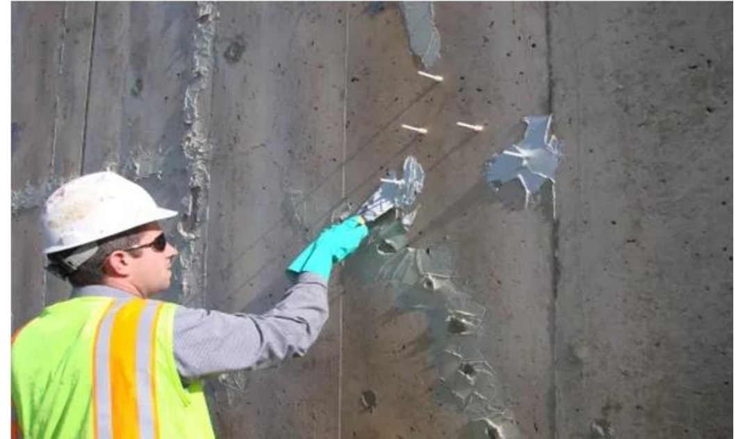
Figure: Applying Epoxy to the Cracks
