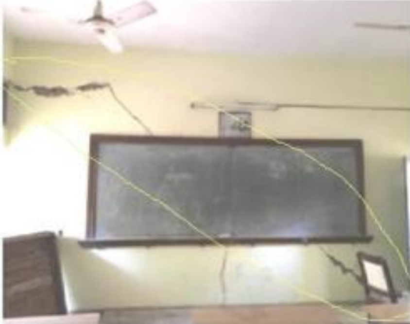
Figure 1: Short Wall of classroom 16 (political block)
