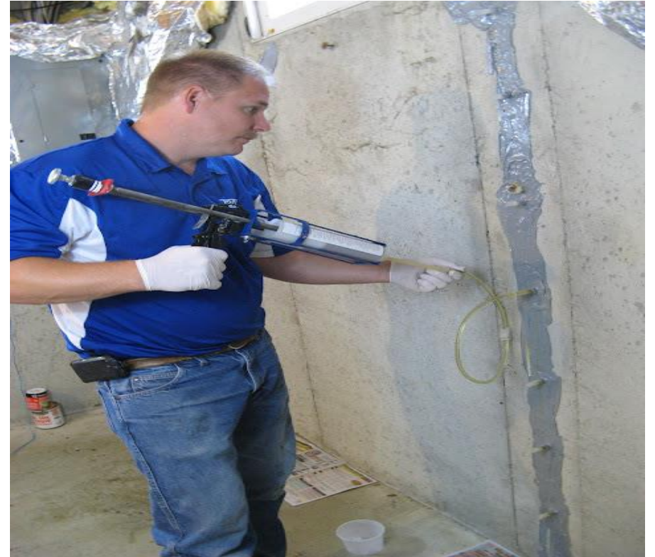
Figure: . Epoxy Injection Method(Source:Ascelibrary(n.d.):Online) https://ascelibrary.org/doi/abs/10.1061/(ASCE)1084-0680(2008)13%3A4(175)
