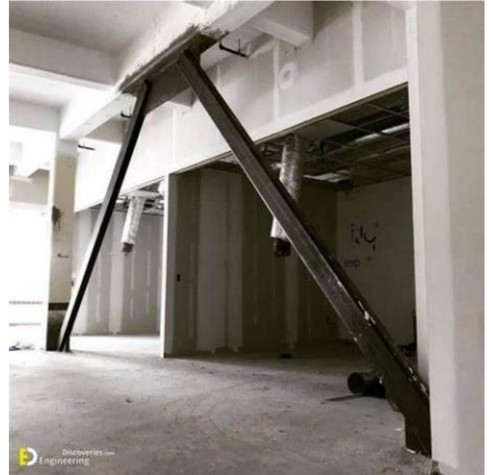
Figure: Steel Bracing(Source:Engineering Discoveries(n.d.): Online)
