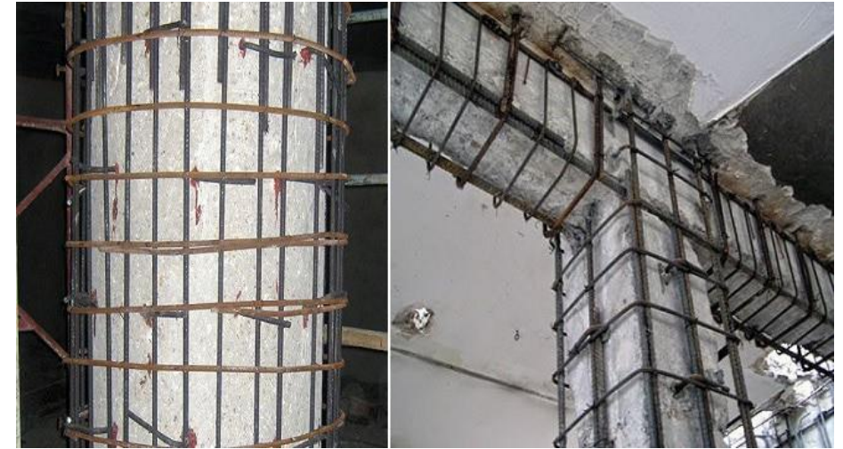
Figure:Jacketing(Source: Civiconcepts(n.d.):Online https://civiconcepts.com/blog/retrofitting
