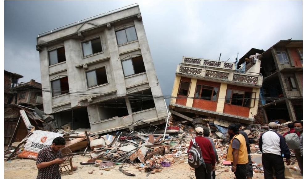
Figure: Earthquake effect(Source:The Guardian(n.d.):Online) https://www.theguardian.com/cities/2015/apr/30/nepal-earthquake-disaster-building-collapse-resilience-kathmandu
