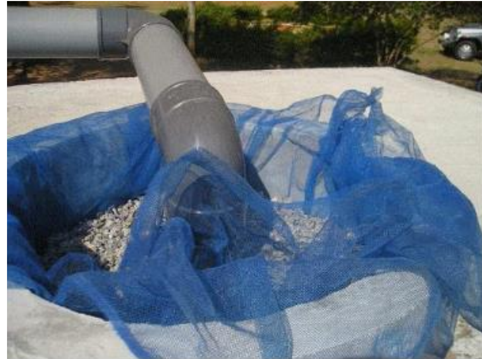
Figure: Photograph of Typical Filter in Rainwater Harvesting (Source: The Constructor: Building ideas. (n.d.). ):Online https://theconstructor.org/water-resources/methods-rainwater-harvesting/5420/#google_vignette
