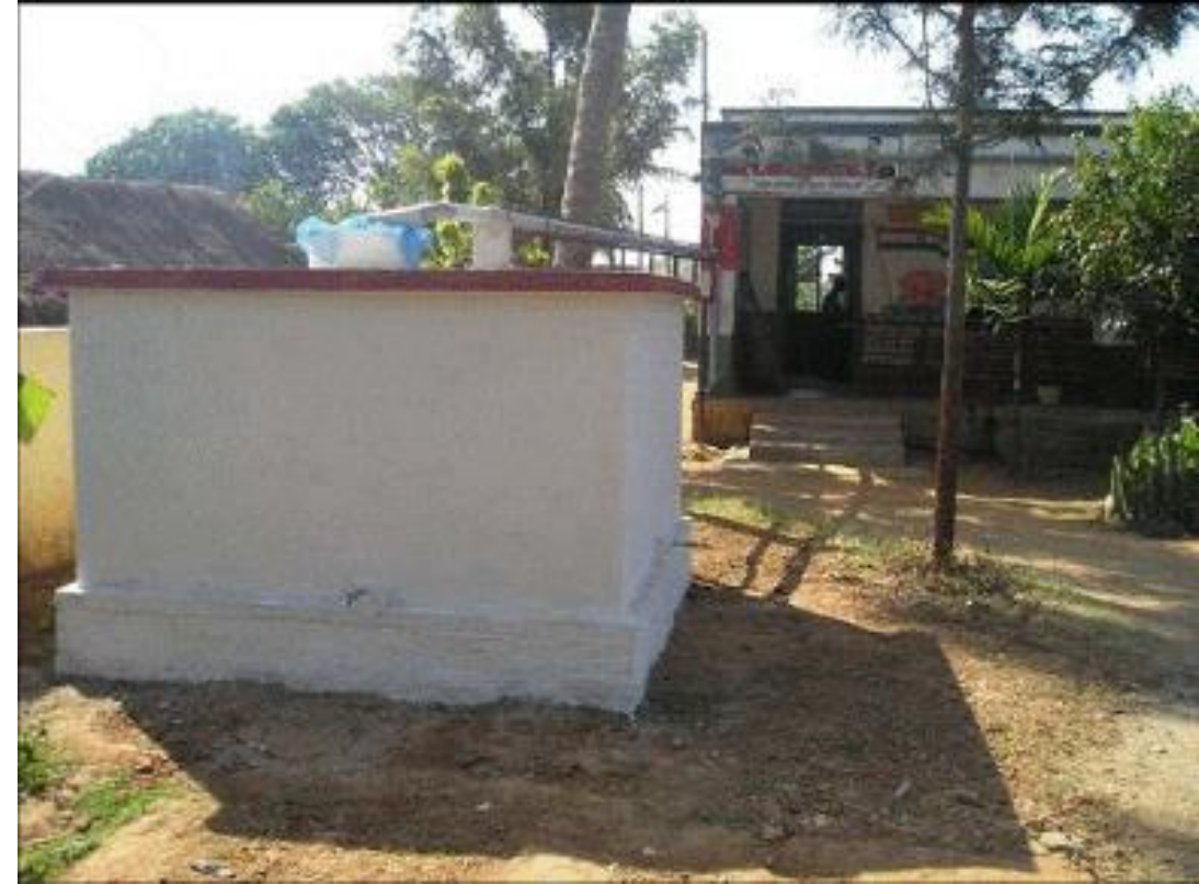
Figure: A storage tank on a platform painted white(Source: The Constructor: Building ideas. (n.d.). ):Online
