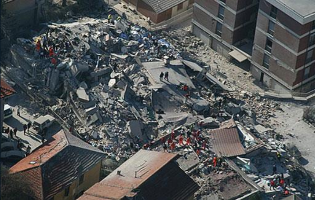
earthquake damage in Italy that killed several hundred people; (Ho/Reuters/Newscom)
