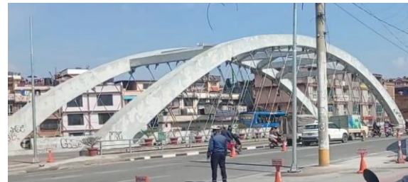
Bijuli bajar concrete arch bridge, Kathmandu.
