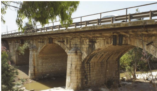
Masonry arch bridge
