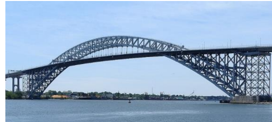
Bayonne bridge between New York and New Jersey (Steel arch bridge)
