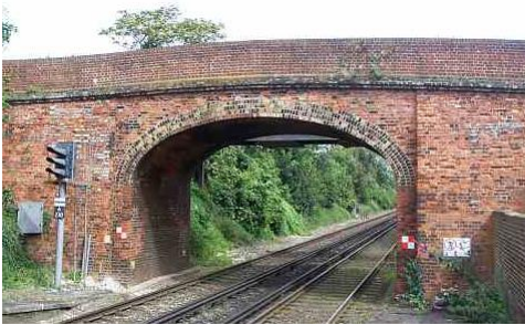
Bridge 812 at Birchington-on-Sea (semi-elliptical arch)
