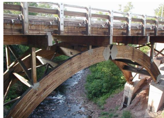
Eagle river timber arch bridge
