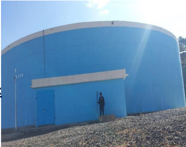
Service reservoir: Addis Ababa
