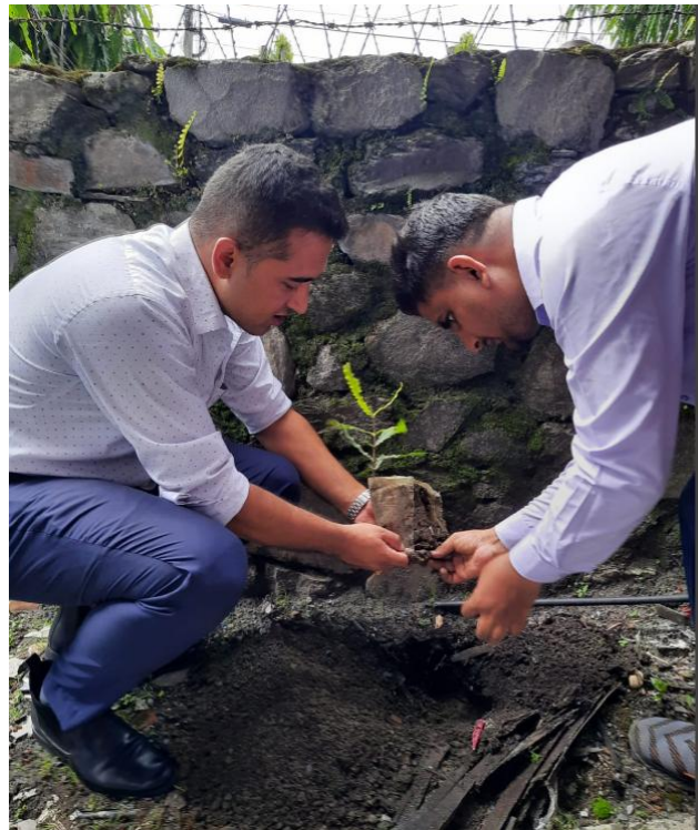
Figure 12: Retaining Wall (©Sunil Rakhil,2024)
