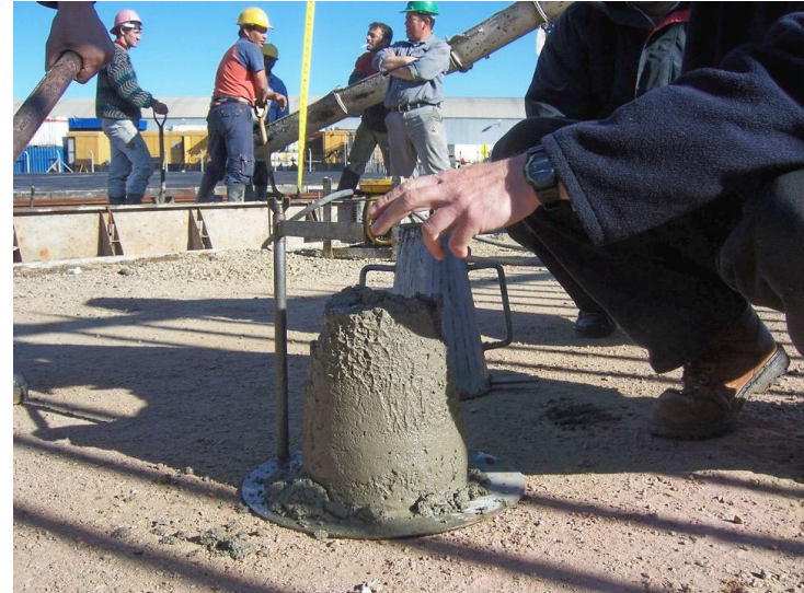
Tano4595 (2006). Measuring the slump of the concrete [Photograph] . Wikimedia Commons. https://commons.wikimedia.org/wiki/File:Cono_de_Abrams_05.jpg
