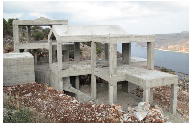
Macrolepis (2008). Unfinished concrete building [Photograph]. Wikimedia Commons. https://commons.wikimedia.org/wiki/File:Unfinished_concrete_building_-_panoramio.jpg
