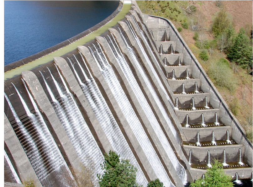
OLU (2008). Clywedog Dam [Photograph]. Wikimedia Commons. https://commons.wikimedia.org/wiki/File:Clywedog_Dam_-_geograph.org.uk_-_784825.jpg
