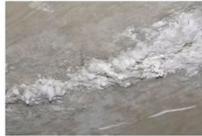
Sulfate attack on concrete. Source: CTLGroup Qatar. (2019))
