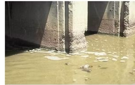
Sulfate attack on concrete. Source: CTLGroup Qatar. (2019))
