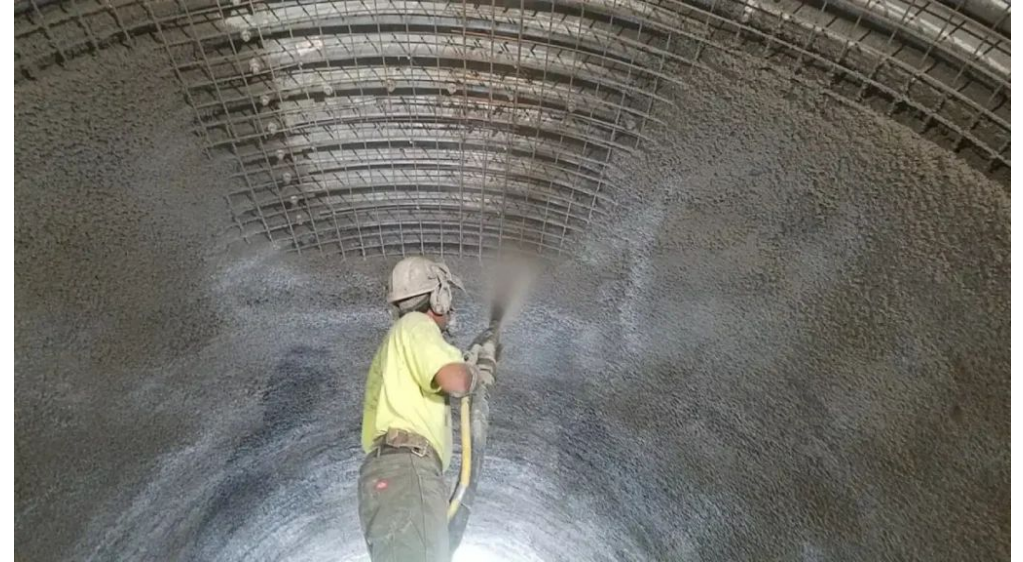
Shotcrete as final tunnel lining Source: Thompson, A. (n.d.)
