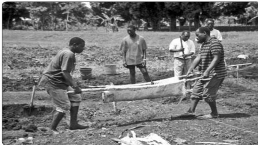
Figure 2.2-5. A two-person stretcher works very well for moving soil from the excavated area to the embankment area, especially in heavy clay soils.
