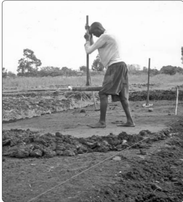
Figure 2.2-6. Dyke construction is done in layers about 20 cm thick. Each layer is well compacted before the next layer is added.
