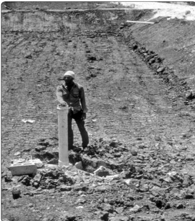
Figure 2.2-7. A PVC standpipe being installed in a new pond. With the standpipe in the vertical position the full pond will have a water depth of approximately 1 m.
