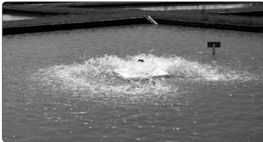
Figure 4.7-5. An electrical aerator.
